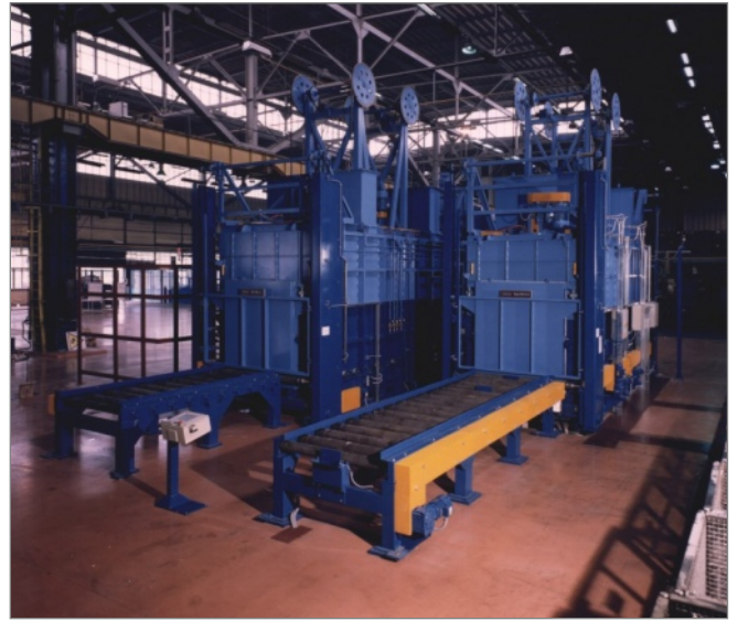
Solution heat treat furnace, front view
